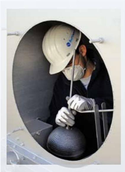
BAC Balticare offers a choice of preventive inspection and electro-mechanical maintenance programmes in accordance with BAC's Operating and Maintenance Instructions. These include inspection of the general condition of the BAC unit with particular regard to evidence of corrosion or scaling of vital heat exchange and internal surfaces caused by inappropriate water treatment.
