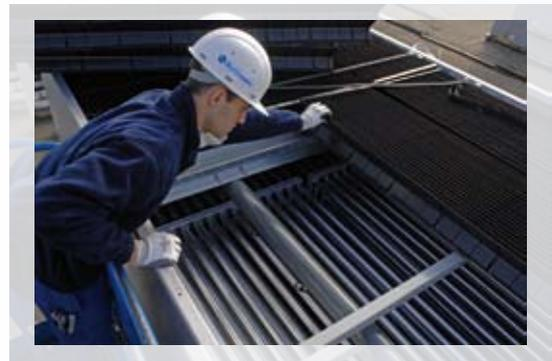
In addition all work carried out will be accompanied with a report by the BAC Balticare service technician which records the work done and makes suggestions for other replacement parts or remedial measures to restore optimal operational and safety levels. This will ensure the BAC equipment is well maintained to maximise system efficiency and minimise operating costs and energy usage.
