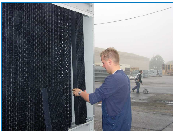
Remove combined inlet shields
