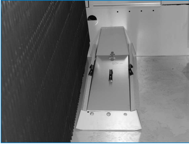
Cold water basin and basin strainer
