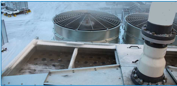
Hot water basin and optional distribution pan covers
